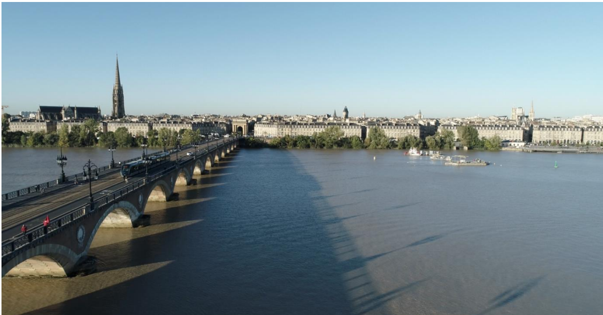
Figure 1: View of SEENE OH Test Site. Credit: VISUAILES
